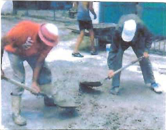
The cement was mixed on the ground, then shoveled into wooden and re-bar structure supports.
