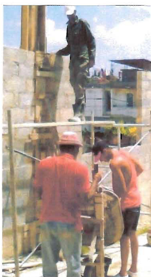
With the perimeter support posts complete, the cement blocks were laid, then smooth coated.
