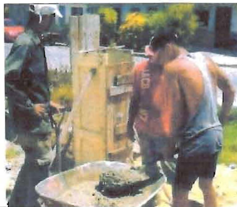
The cement was mixed on the ground, then shoveled into wooden and re-bar structure supports.
