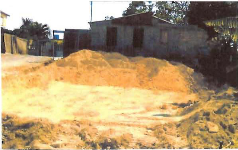
Havana, Cuba: The ground was cleared and leveled. Then a trench for the perimeter wall was dug.
