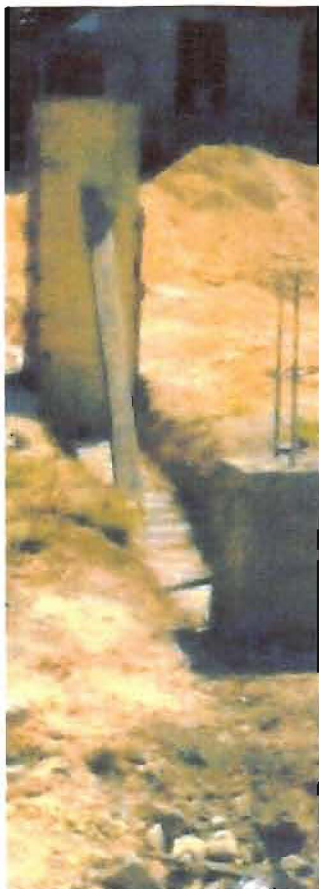
With the perimeter support posts complete, the cement blocks were laid, then smooth coated.
